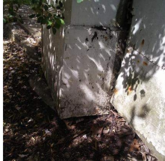
Foundation unknown, concrete pad only visible
