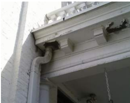
Soffit repair, clean, replace rotted wood
