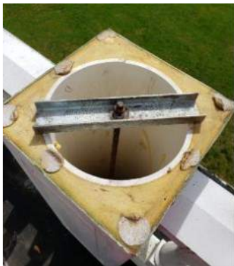
Repair loose caps
