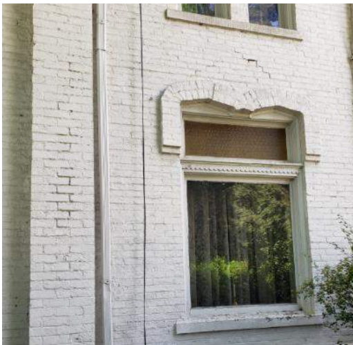
Tuckpointing/brick repair
