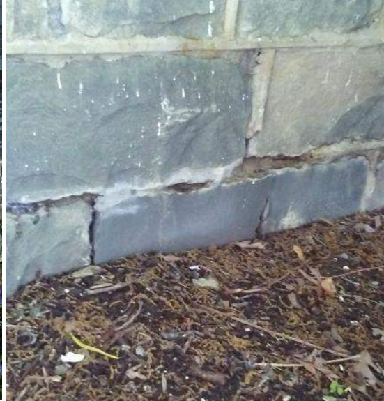
Foundation mortar repair
