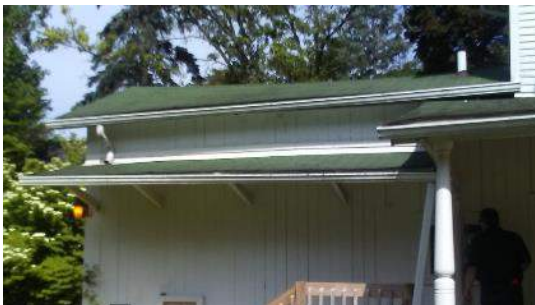
Replace shingled roof
