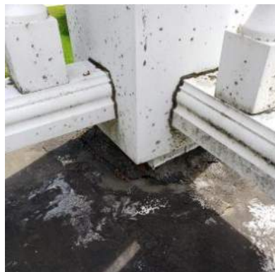
Miscellaneous flashing repairs, clean PVC panels.
