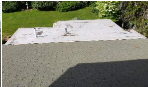
Replace membrane roof.
