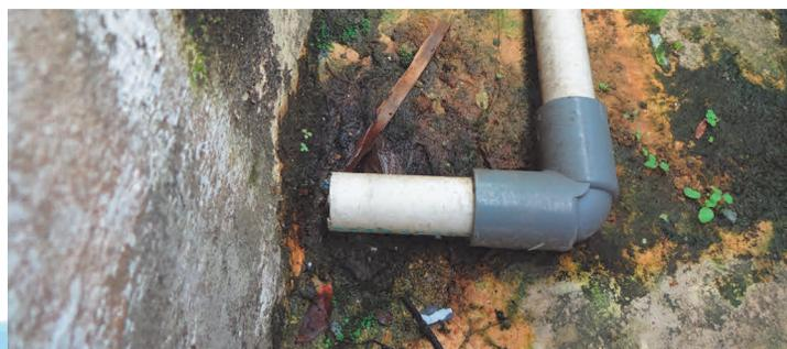
Never reroute sanitary drains on your property without verifying their connection to a sanitary sewer system. If a sewer pipe is mis-connected to a storm drain system, this is an illicit connection and is harmful to water quality.
