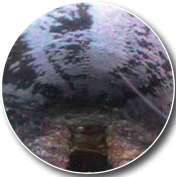
View of FOG build-up inside sewer pipe
